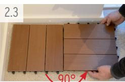
Rotate the next deck tile anti-clockwise at a  $90^\circ$  angle.
