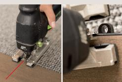
If the tiles have to be cut, please use a jigsaw. It can be sawn through the tile and the support material. Please remove the loops at the outside edges before laying the last row of tiles.
