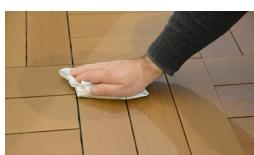
... apply a thin layer of Resysta Top Care Oil onto the surface.
