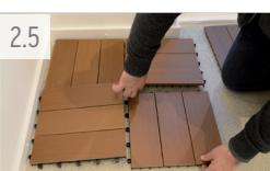
At every 4th tile, it is necessary to lift the two subsequent tiles to slide the flaps under the preceding tiles.
