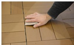
If this procedure should not be sufficient, use 80 - 100 grit sandpaper. Sand lightly. NOTE: If sanding is performed to remove stain, re-oiling may be required.
